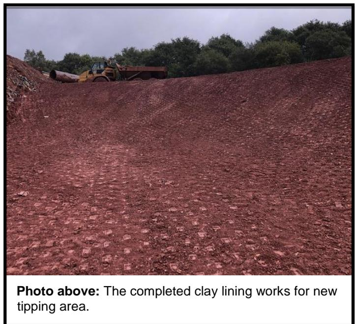
**Photo above:** The completed clay lining works for new tipping area.
