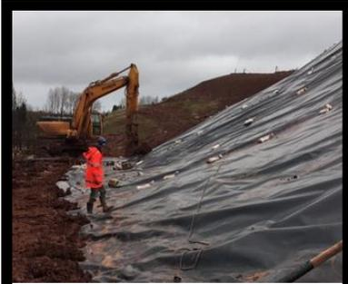
**Above:** Temporary geomembrane capping on the flanks of Cell 3 (near to the site entrance)
