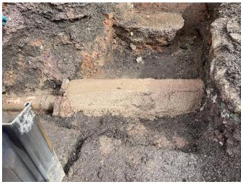
The concrete blinding in the Stourport Road (Area 4 and 3) is now complete. Work has begun on pressing the trench sheets into this section and this continue into next week.
