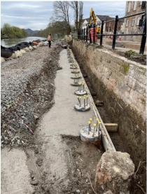
Where the existing access steps have been removed next to the quayside wall near to the junction of Stourport Road and Kidderminster Road, the ground is to be excavated, refilled, and compacted to ensure this creates a suitable working area.
