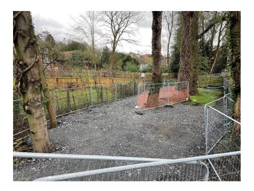
Cadent Gas have finished the gas diversion works as well reinstating the section adjacent to the bridge (Area 1). The reinstated ground will now need to be assessed for suitability for future piling works. Cadent Gas will move in the coming weeks into the Pleasant Harbour section (Area 0) for further diversion works there.
