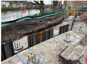
We have excavated a section of the previously laid concrete blinding in Area 5, in order to lay the rising main. The intention is to then install that pipe and associated puddle clay stank and flange in preparation for pile capping. We have also encased an existing foul drain in Area 5 to protect the pipe from potential damage where it passes beneath the capping beam.
