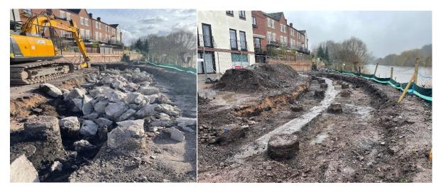
All the piling around Millside Court is now complete, but some of those piles have required a casing, which will need to be cut down to the required level. This week we have been exposing these casings in preparation for future works.
