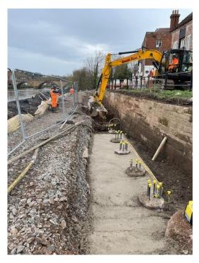
Where the blinding and piling is in place in Area 5, we have now installed trench sheeting. This will allow us to reduce seepage through the defence when in place. Where the trench sheets are in place the next stage will be to burn out the sections necessary for the capping beam to follow. This will also include welding studs into these sections for reinforcement.
