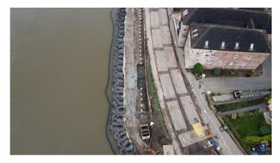
Further works are being completed in the Pleasant Harbour House (Area 0) section of the site to prepare the area as an access for the piling phase. Fencing is being put in place as well as root protection track matting, followed by access track and piling pads to build a route through for the Area 0 works.
