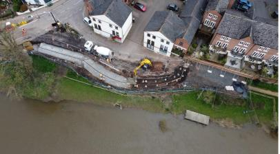
Severn Trent Water (STW) have confirmed that it is safe to remove the previously unknown and unused manhole chamber in area 5. The removal is required because the manhole chamber is located in the middle of our flood wall alignment, and it would not be viable to work around it. In order to undertake removal safely, we need to install trench sheets to provide stability of the excavation walls.
