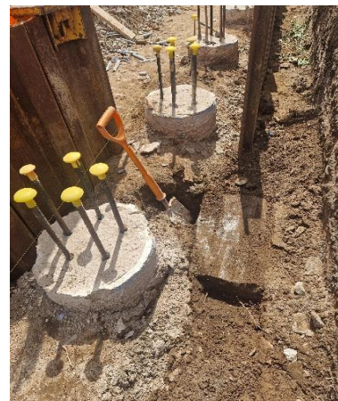
Engineered trench sheet solution
