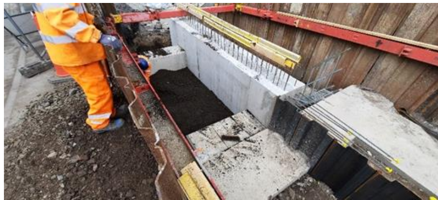
Backfill and compaction Area 4
