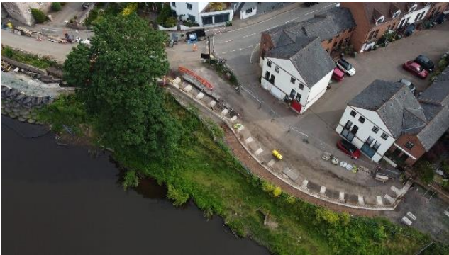
Millside Court backfilled section
