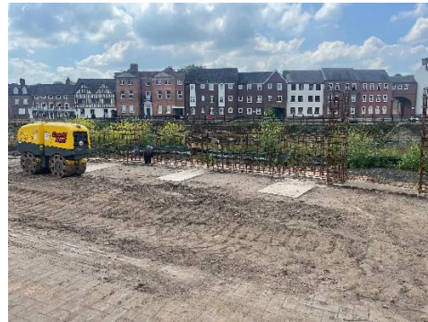
Compacted ground at Millside court
