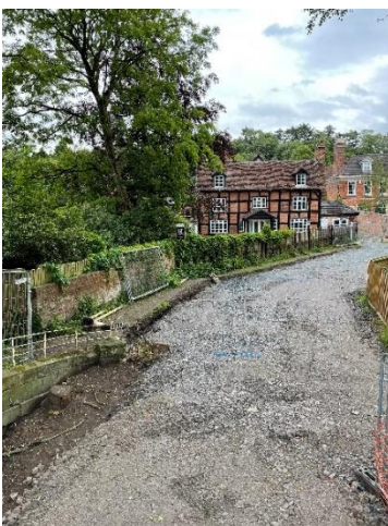
Area 0 piling pad
