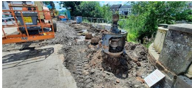
Installation of pile castings in Area 2
