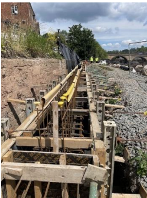
Shuttering/reinforcement Area 4
