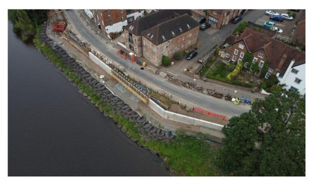
Much of the Area 3 (Stourport Road) wall is in place, with a short section as it moves into Area 2 still to be complete. The piles are in Place in Area 2 (Stourport Rd/Kidderminster Rd junction) with the piles due to be cropped and cleaned in the coming days. We crop the piles in order to prepare them for pile capping stage, and the pile capping is the structure we put in place on top of the piles in order to connect and create strength in one flood defence structure.
