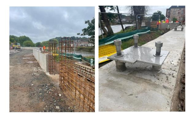
The concrete core wall in Area 4 (Stourport Road, Millside Court end) is complete, with only some drainage work to undertake. This drainage work is to ensure that flood defence doesn't impact on the current surface water drainage regime in the area.
