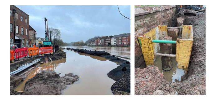
In Area 5 (Millside Court) the flood wall core is now in complete. The fittings for the glass wall top and reinforcement for the flood gates are in place ready to move to that stage of the scheme.
