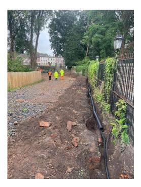
With the piling in place the next stage will be putting in the trench sheets, exposing and cropping the piles and putting the concrete blinding in place. This will allow us to put the capping beam in place and move on to the steal re-enforcement and flood wall concrete core.
