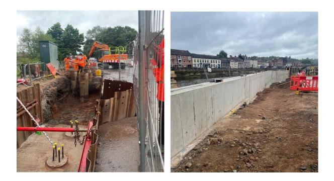
All the piling is complete in Area 1 (Adjacent to the bridge) and the ground compacted. As with all the piles throughout the scheme these will have to go through integrity testing before the next stage of the flood wall build.
