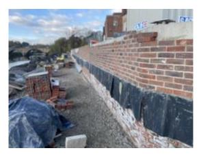
The copping stones are due to go on top of the wall soon. They are made of reconstituted stone that matches the colour and texture of the new sandstone found on the Grade I-listed bridge.
