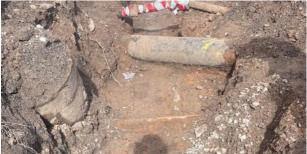
As well as removal of services not in use, we will also be taking out a section of an extinct brick culvert in preparation for the piling and capping beam that will be in place in that location.
