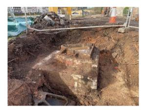
We have removed most of the coping stones from the quayside wall, in preparation for continuing the work along Stourport Road.
