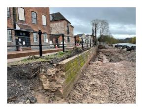
Ahead of the next phase of piling works, we have undertaken vegetation clearance at the rear of Pleasant Harbour House to prepare the area for construction plant access and deployment of piling mats.
