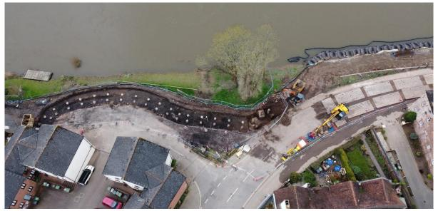
During the excavation, a masonry manhole chamber was uncovered that we were previously unaware of. We are working closely with the Severn Trent Water Asset Protection team who are helping us with amendments to current capping beam design.
