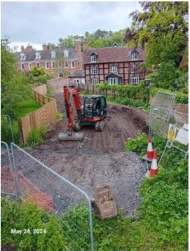
Work on excavating the old wall that stood next to the footpath at Pleasant Harbour House (Area 0) was completed last week. Now this is done, we will be removing topsoil and putting down stone, in preparation for the piling mat.
