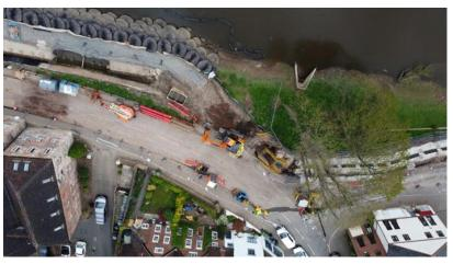
We have been installing sheets and frames around the Severn Trent manhole. Next week we put down the blinding in this area. This will all enable us to reduce the height of the manhole cover in a safe and efficient manner.
