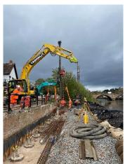
Cadent Gas have revisited the diversion works in the area in front of the bridge. This work has had to be re-excavated and compacted due to complications in the compaction process. This work has also impacted on the programme of works at Pleasant Harbour, with alteration to the traffic management moving from the river side of the road to the pleasant harbour side of the carriageway now planned for next week. This should be in place from early next week for a period of 3 or 4 days.
