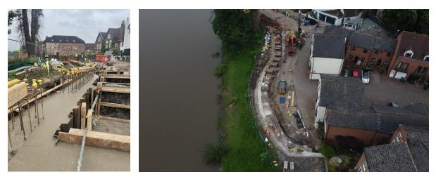
The manhole chamber at the junction of Stourport Road and Millside Court (Area 5/4) has been lowered to the required level. Blinding has been placed and is now ready for reinforcement and shuttering to construct the capping beam.
