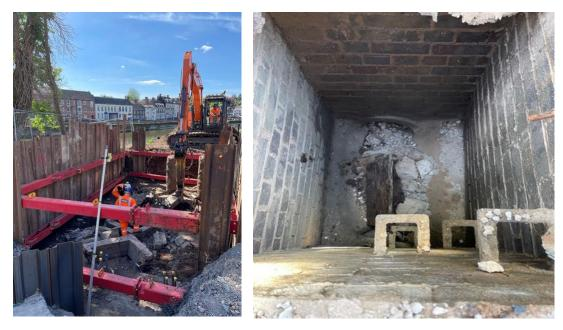
Redundant gas and water pipes on Kidderminster Road (Area 2) and adjacent to the bridge (Area 1) have been removed. Piling has recommenced on Kidderminster Road (Area 2) and the piling mat construction is progressing adjacent to the bridge (Area 1) in preparation for future piling works.
