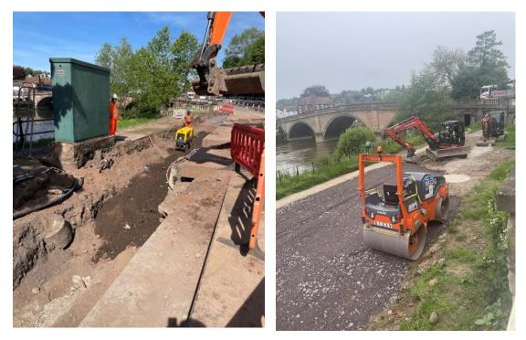
In Area 2 piling mats have been laid down and piling has begun this week. Although piling work is progressing, with 97 piles installed to date, and 92 still to install, we have more recently encountered a harder section of rock at a higher level and as such piling is a little slower at this time.
