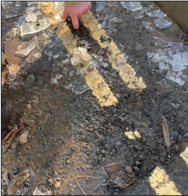
Figure 35: Loose aggregates in the dressing layer no longer bonded to the pavement structure.
