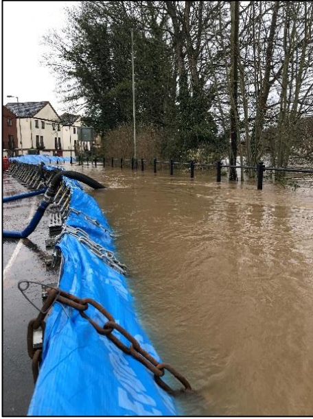
Figure 4: Pump discharge hoses can be observed crossing the barrier.
