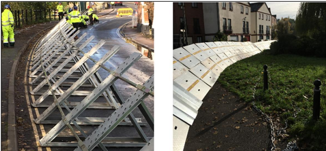
Figures 2 and 3 show the modular nature of construction of the system with legs, plate bars and plates.
