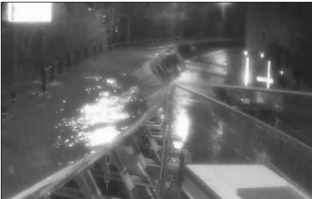
Figure 25: EA Remote Camera photograph showing inward movement of a section of barrier at the centre of the image at 23:34.
