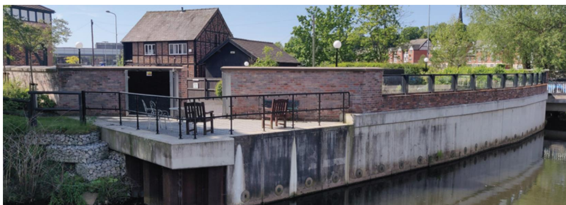
View of new flood defence in Northwich, Cheshire (Photo by IBS)
