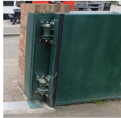
Upton-upon-Severn flood defence flood gate
