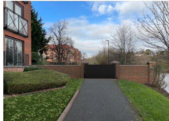
Yarm Flood Alleviation Scheme flood gates (Pictures from Environment Agency)
