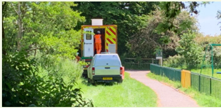
Preparing for ground investigation works
