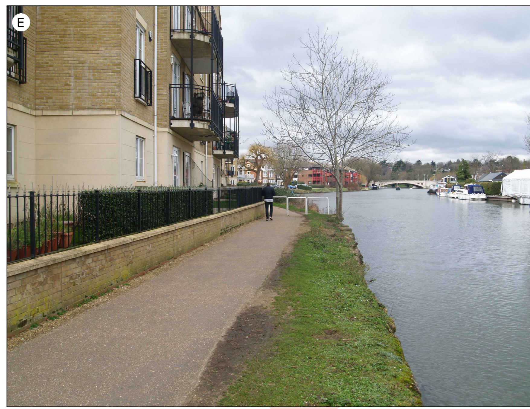
Brick finish at Regents Riverside - smooth, buff coloured face with red engineering brick at the base of the wall
