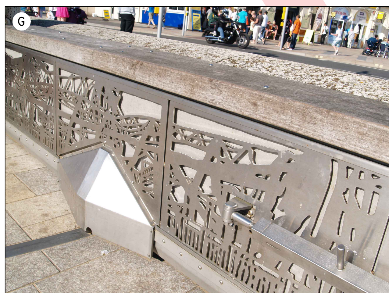
Examples of contemporary flood gate design
