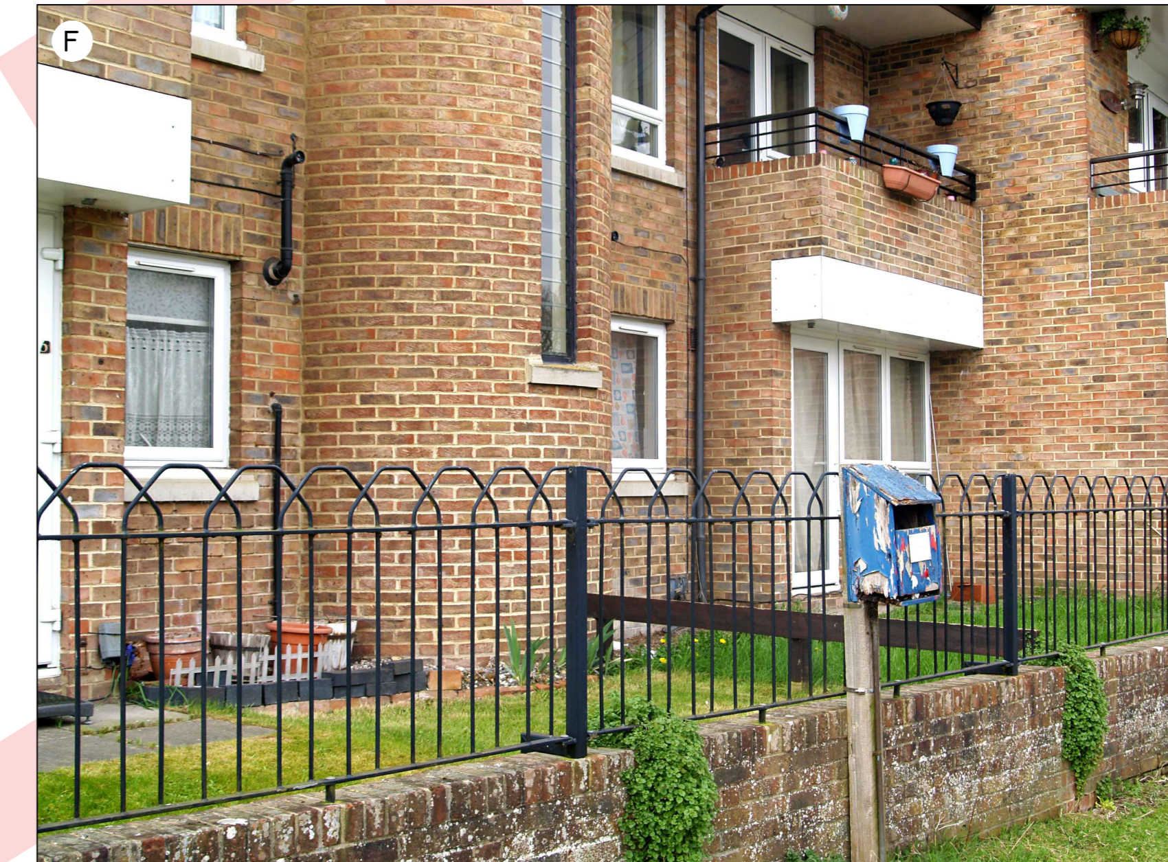
Brick finish at Isis Court - random mix of red and burnt shades with white 'metro-land style' mortar
