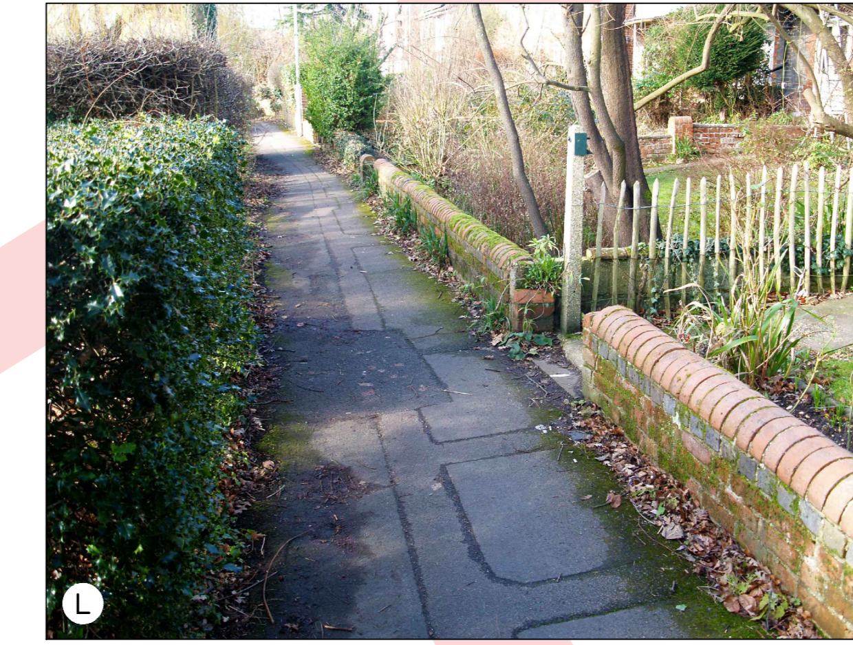
The low walls along the northern edge of Mill Green footpath are an important part of its historical character.
