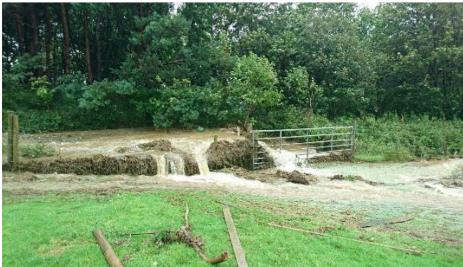
Photograph 1 – Example of a fence creating upstream flood risk
