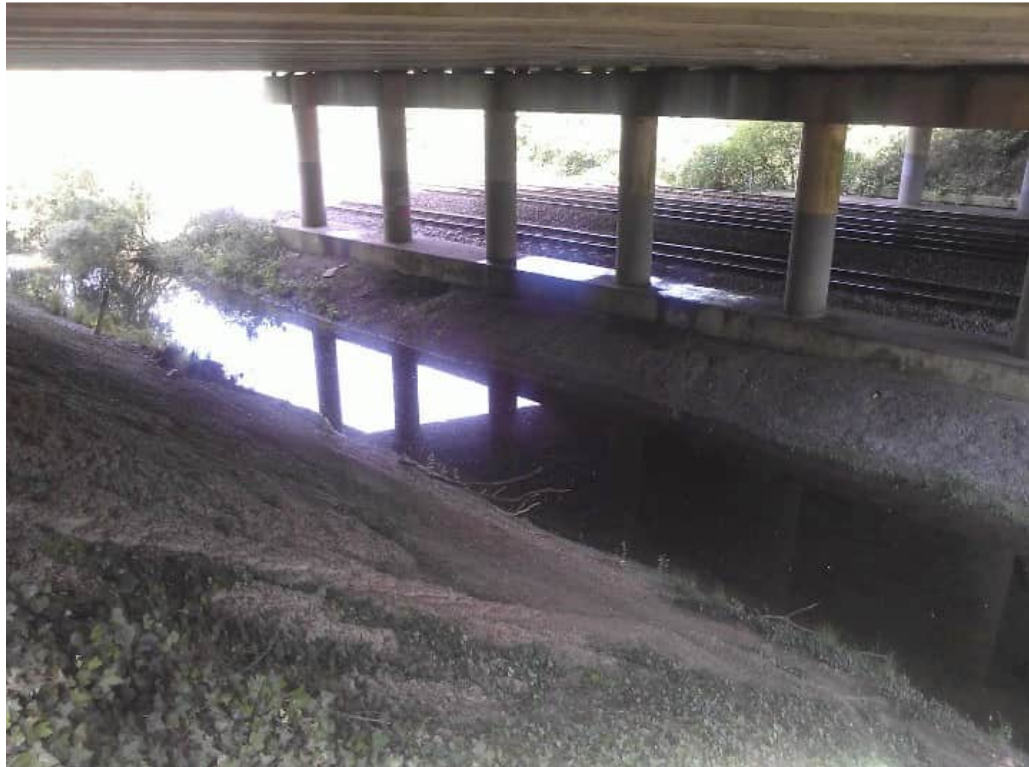
Figure 8 - Underside of the A423 Railway Bridge by Kennington
