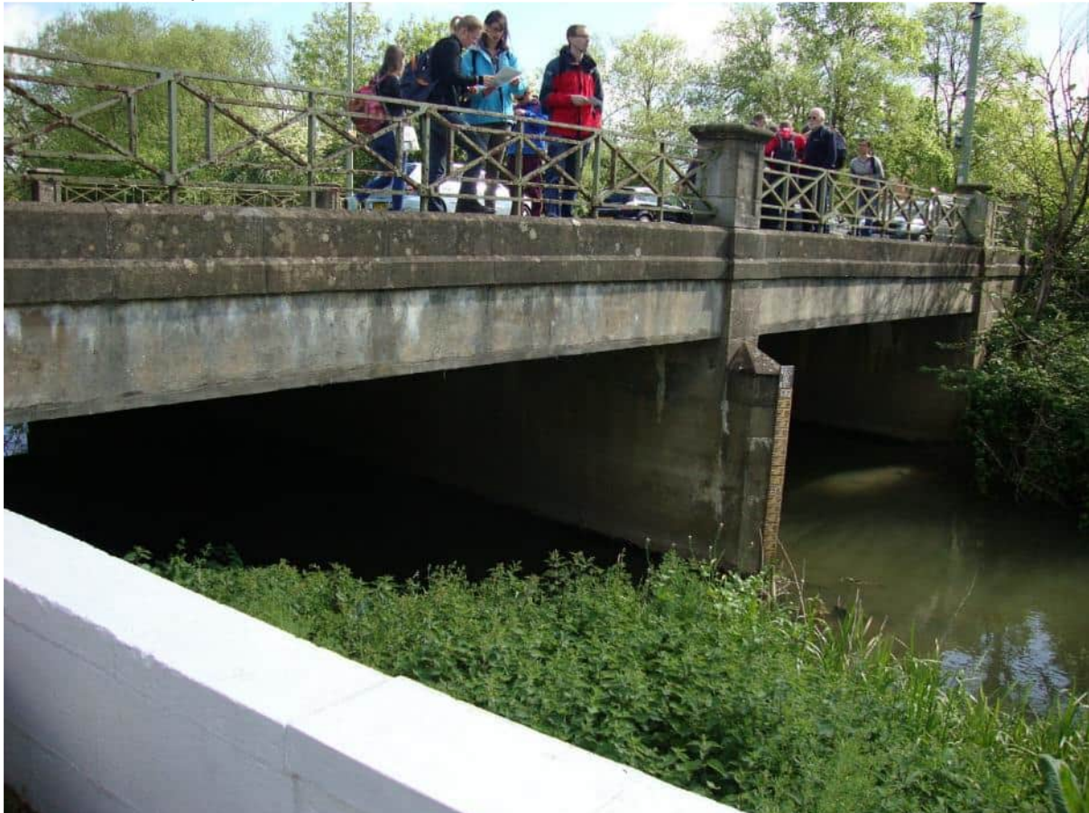
Figure 2 - Seacourt Stream at Botley Bridge
