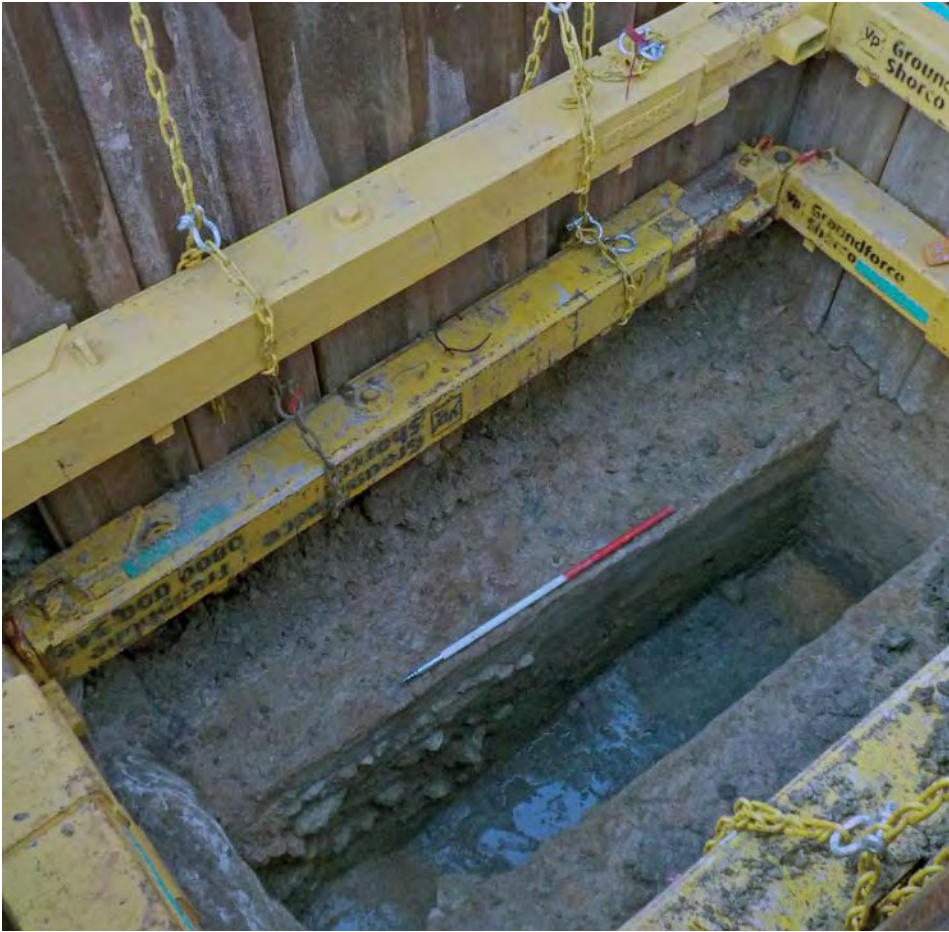
Plate 5: Trench 1 (extension), post excavation, showing linear feature 1091, with kerb stones 1072 toward bottom left of photograph. Scale 1m, looking south-west
