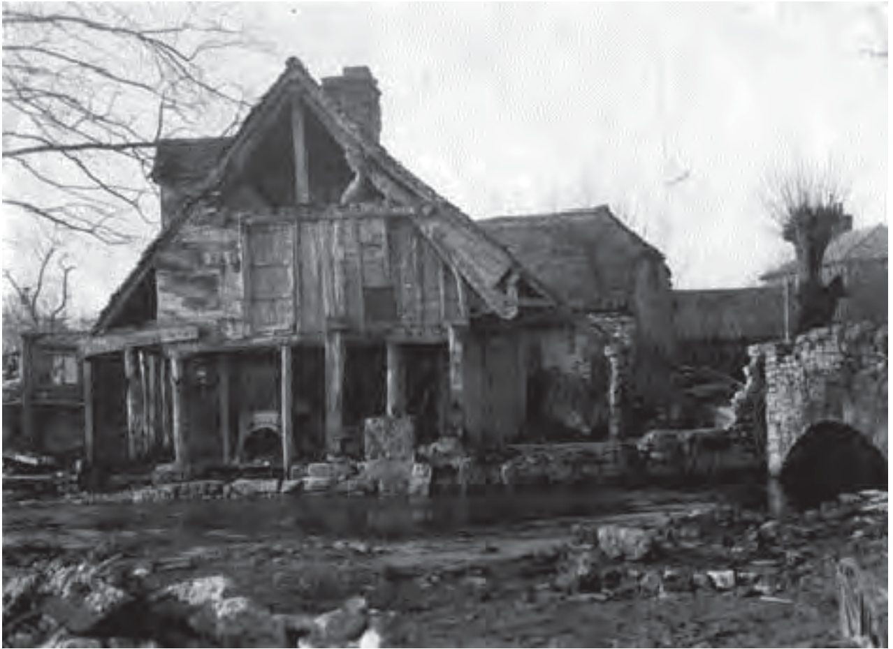
Figure 43: Botley Mill partly demolished during Botley Road widening, 1924 (D262792a)
