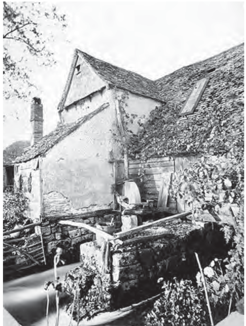
Figure 40: Botley Mill in a state of some disrepair, showing the mill stream and a large whetstone in the foreground, 1875 (Ref. HT1815)
