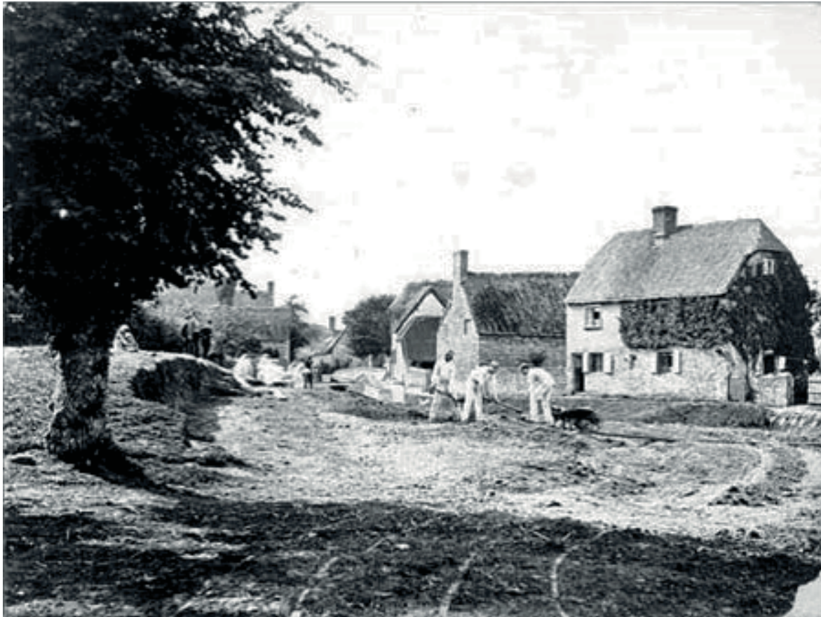
Figure 24: Ruskin Road, North Hinksey, Oxfordshire (1874): the Ruskin road diggers working in the village, with thatched cottage in the background (©Oxfordshire History Centre, ref. POX0113598)
