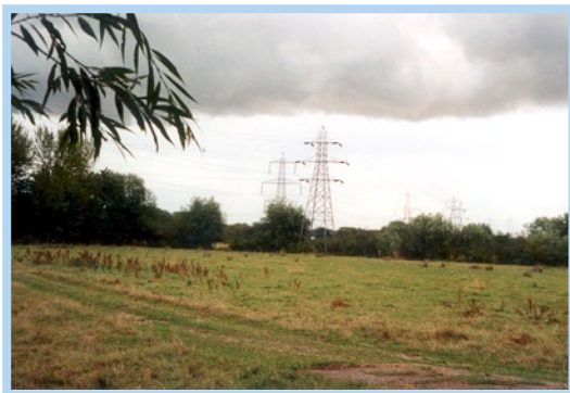
Photo 3: Pylons and transmission lines are prominent.
