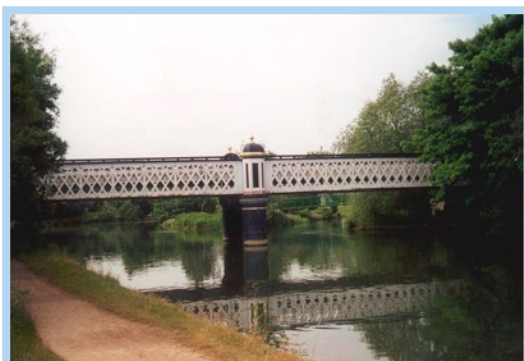
Photo 5: The railway bridge crossing the Thames at Grandpoint Nature Park is a landmark.
