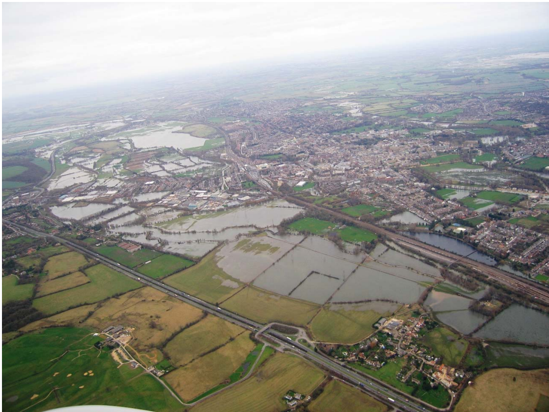
Low level flooding in West Oxford, July 2007
