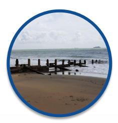
The sea wall and groynes are ageing and reaching the end of their useful life. If nothing is done the timber and concrete groynes will continue to degrade resulting in a loss of the beach material. This would make the sea wall vulnerable to erosion leading to possible failure of the sea wall by 2042. The Isle of Wight Council and the Environment Agency are working together to find ways to reduce coastal erosion and flooding from the sea in Yaverland. The project
