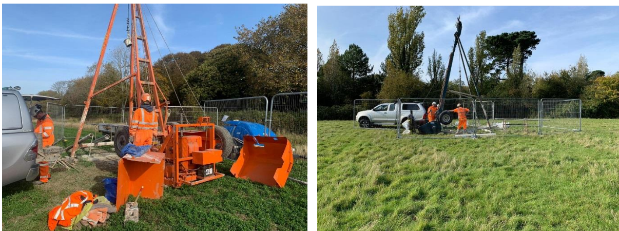
Figure 1: Ground Investigations being completed on Thorney Island in November 2020.
