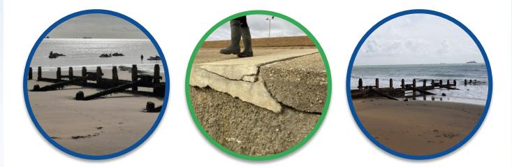
The sea wall and groynes are ageing and reaching the end of their useful life. If nothing is done the timber and concrete groynes will continue to deteriorate resulting in the loss of the beach. This would make the sea wall vulnerable to erosion. The sea wall would rapidly deteriorate causing damage to Esplanade Road (including essential services). Our computer model predicts that...
