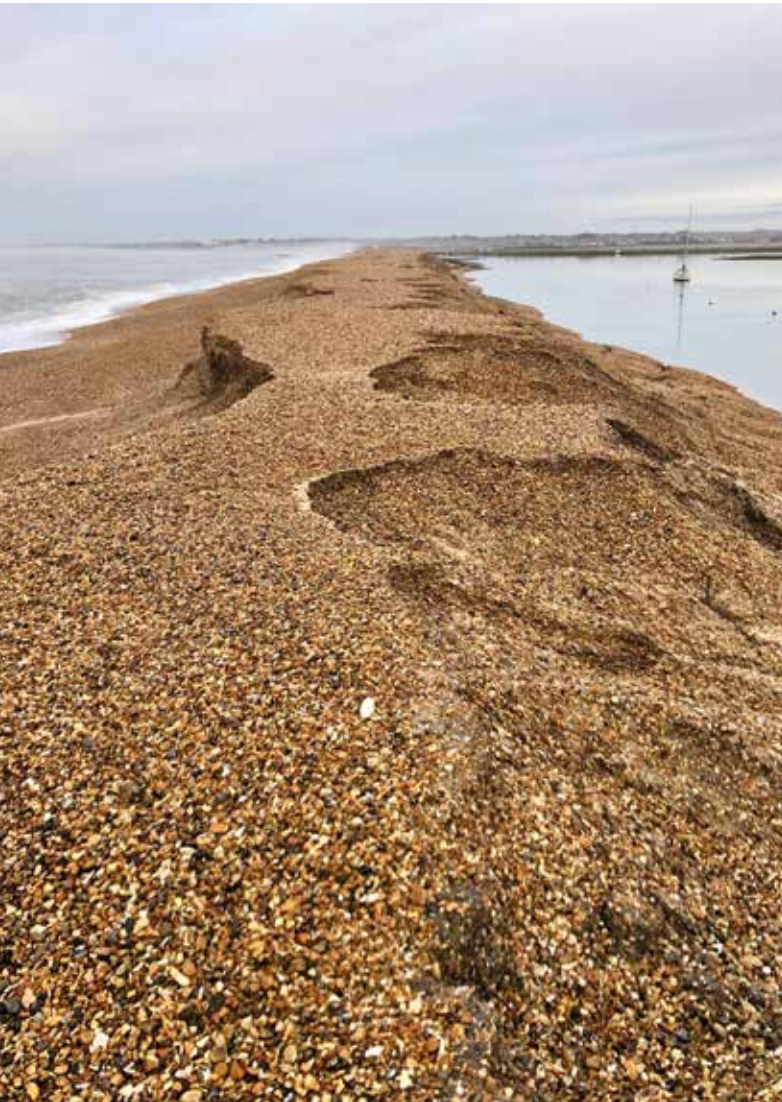
Hurst Spit following a storm in January 2025 Source: New Forest District Council
