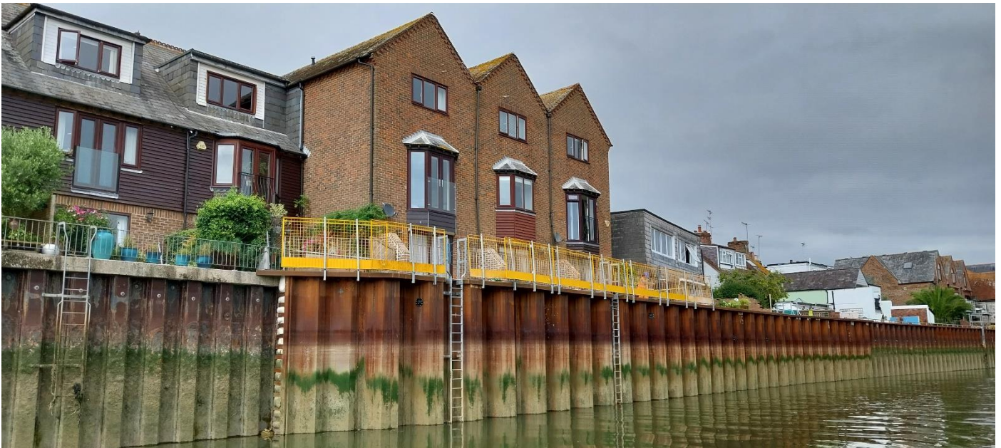
Sheet pile wall from the river
