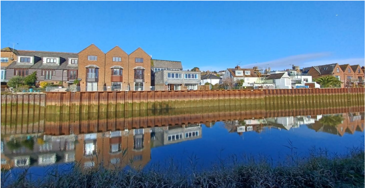
New sheet pile wall
