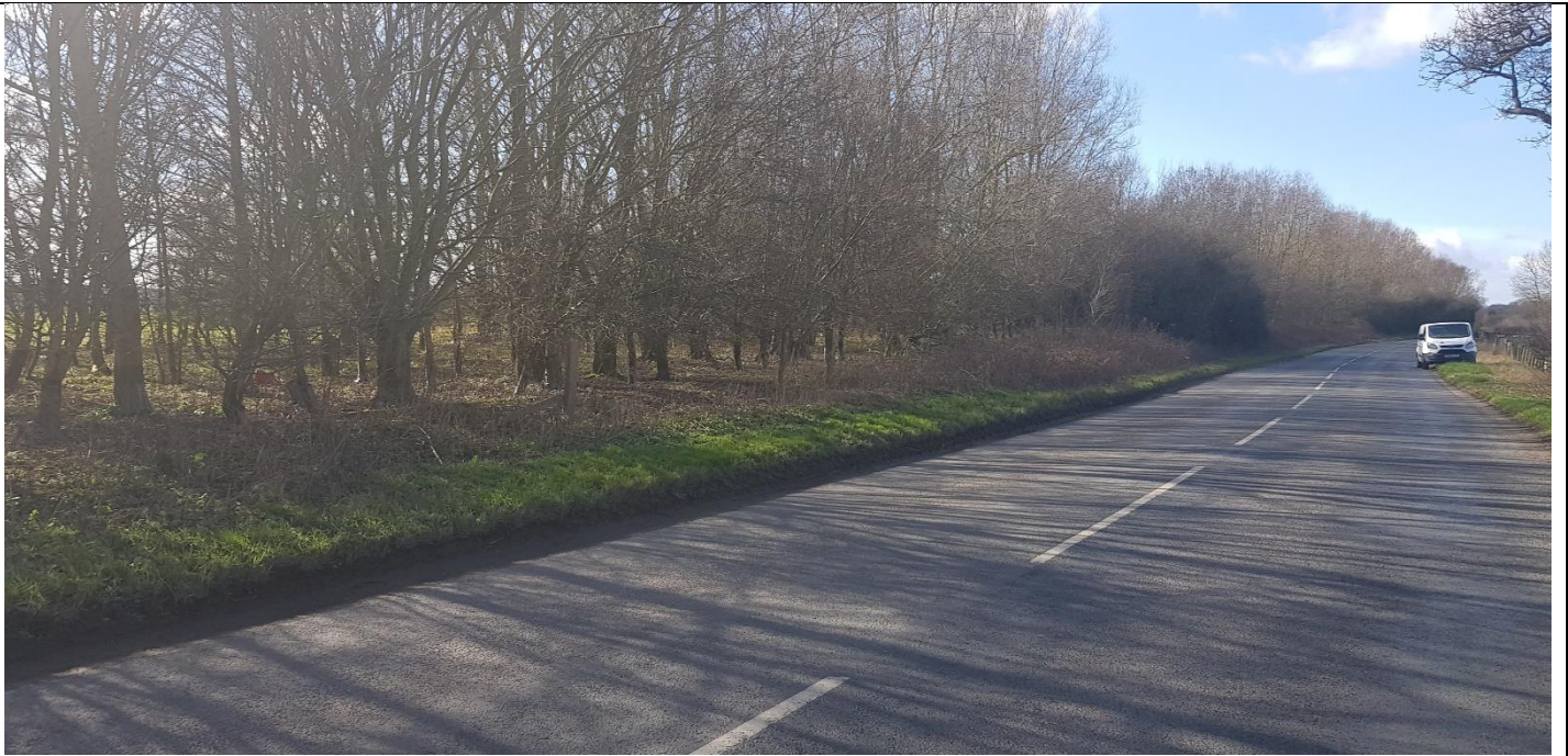
Figure 4: View looking west along the road to the north of the site.
