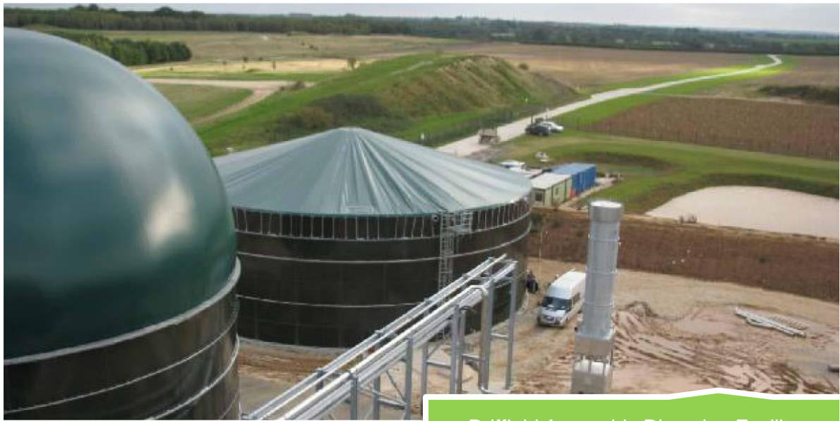
Driffield Anaerobic Digestion Facility
