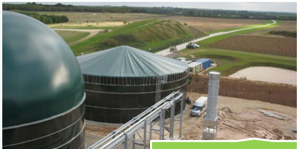
Driffield Anaerobic Digestion Facility
