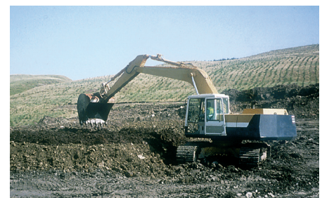
Figure 1 Reinstatement of soil materials using the loose tipping method.
