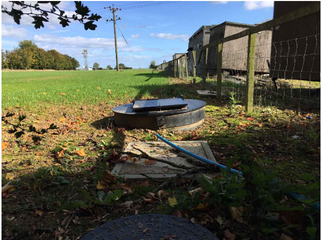
FINAL (WEST) LEACHATE CHAMBER AND ENTRY TO EXISTING SEWER
