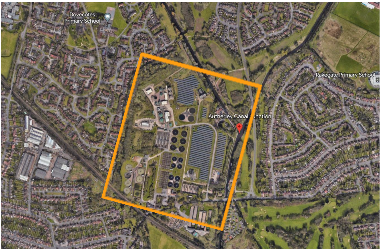
Figure i i Satellite view Barnhurst Sewage Treatment Works
