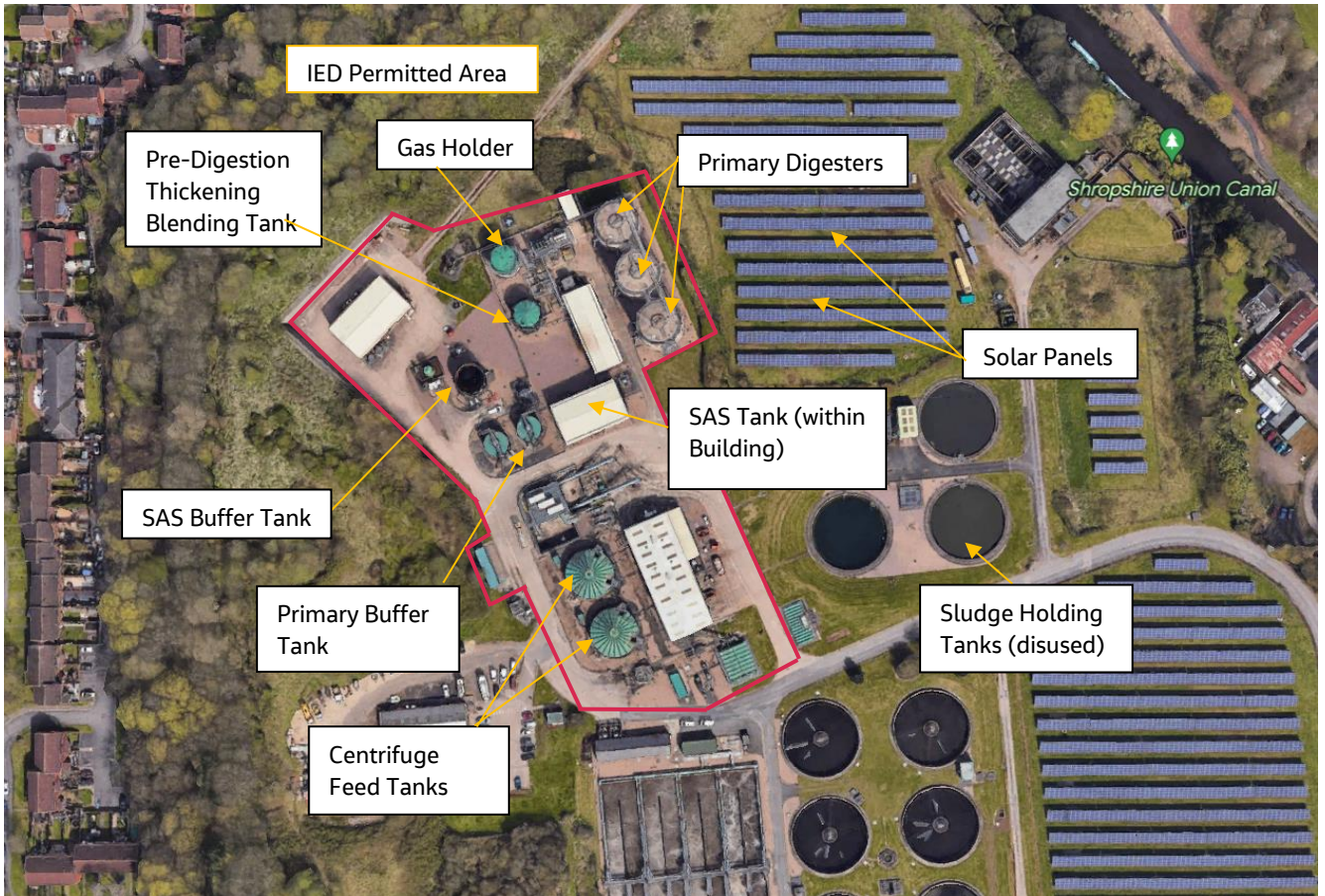
Figure 2.2 Labelled image of Barnhurst Sewage Treatment Works
