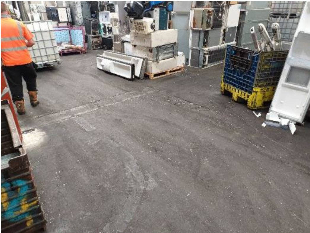
Photograph 27: Example of wear to hardstanding within the internal existing Installation area
