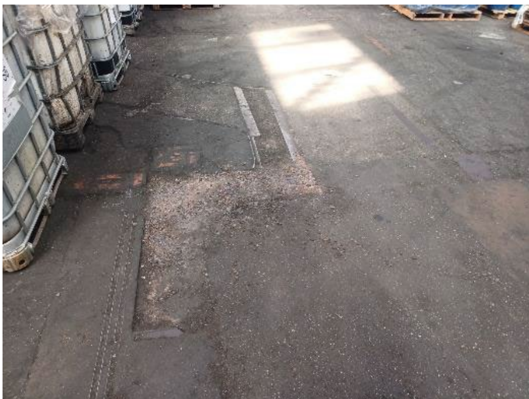
Photograph 6: Example of wear to hardstanding in south of internal Additional Area.
