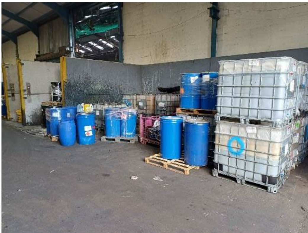
Photograph 13. Chemical Waste Storage Bay with 'sleeping policeman' bunding in existing Installation Area
