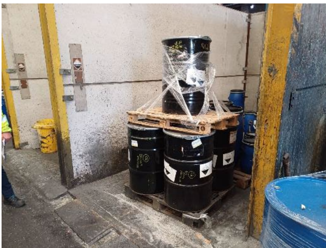
Photograph 13. Chemical Waste Storage Bay with 'sleeping policeman' bunding in existing Installation Area
