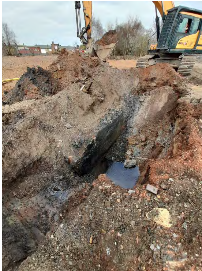
22/03/21 Excavation of validation trial pits around the location of Source 2. The tank wall shown in the picture would be removed in April
