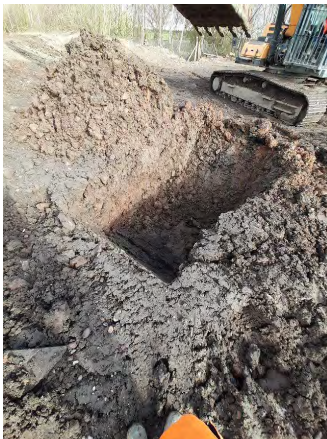
25/03/21 Excavation of validation trial pits around the location of Source 4
