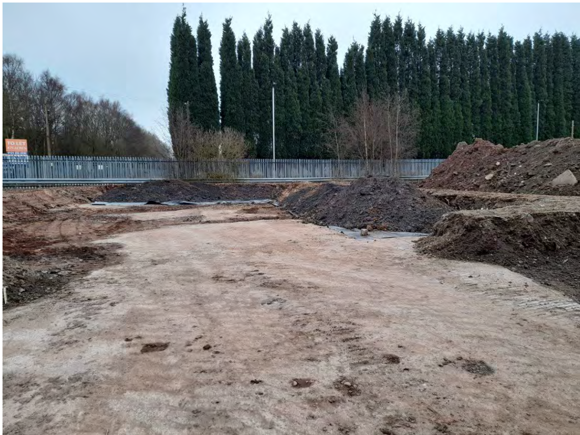
01/03/21 Impacted ground from around HS1 placed in the treatment area, placed upon a impermeable membrane and surrounded by a bund.
