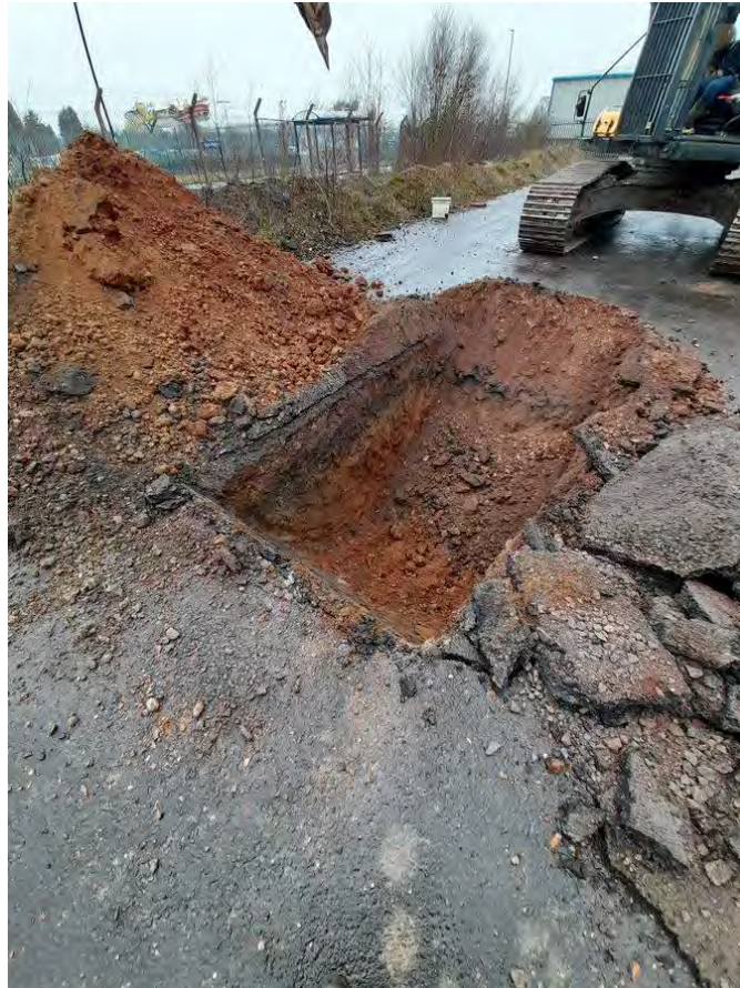
26/03/21 Excavation of western carpark validation samples
