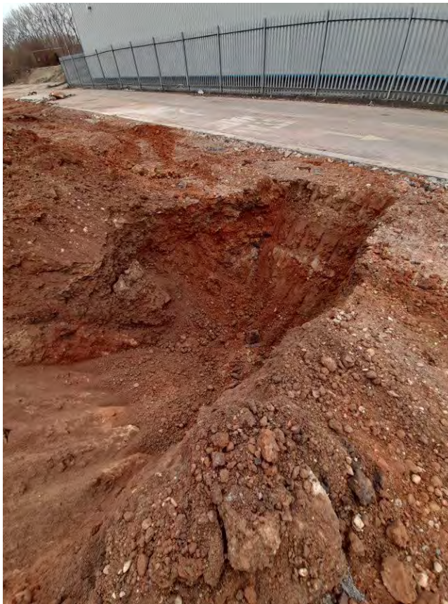
22/03/21 Excavation of validation trial pits around the location of Source 8
