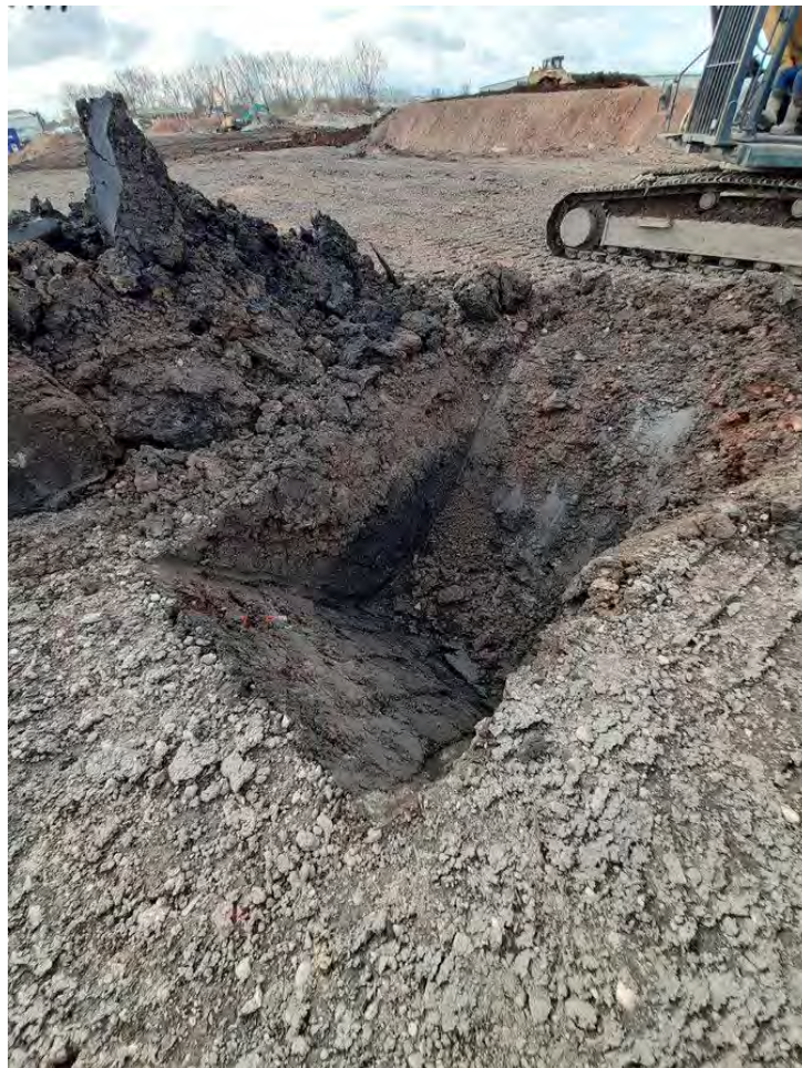
25/03/21 Excavation of validation trial pits around the location of Source 3
