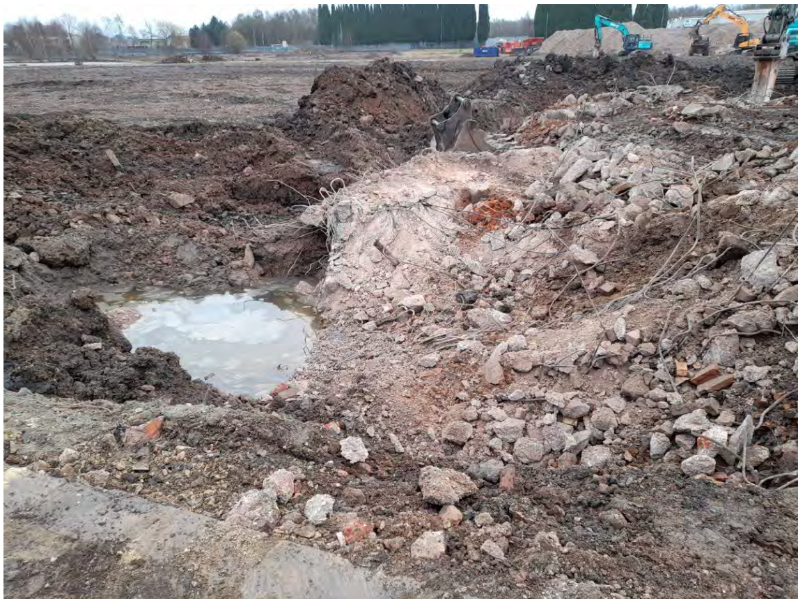
01/03/21 Impacted ground from around HS1 placed in the treatment area, placed upon a impermeable membrane and surrounded by a bund.
