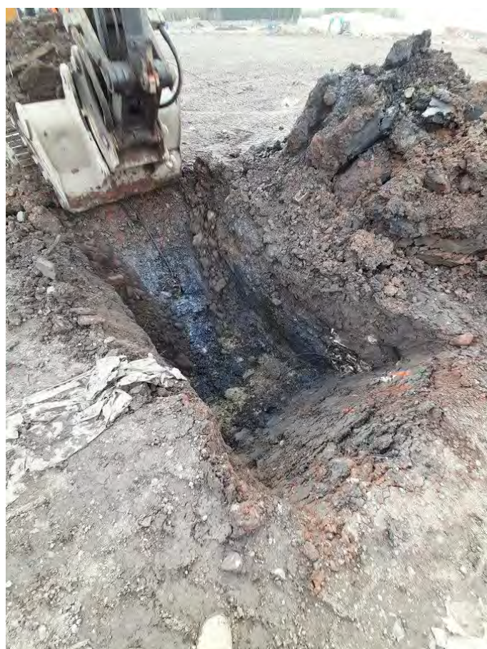
25/03/21 Excavation of validation trial pits around the location of HS3
