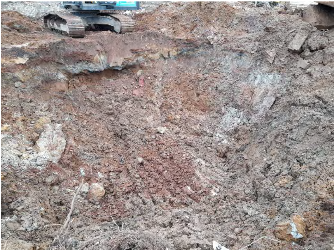
01/03/21 Photo shows the natural clean soils in the base and face of the excavation
