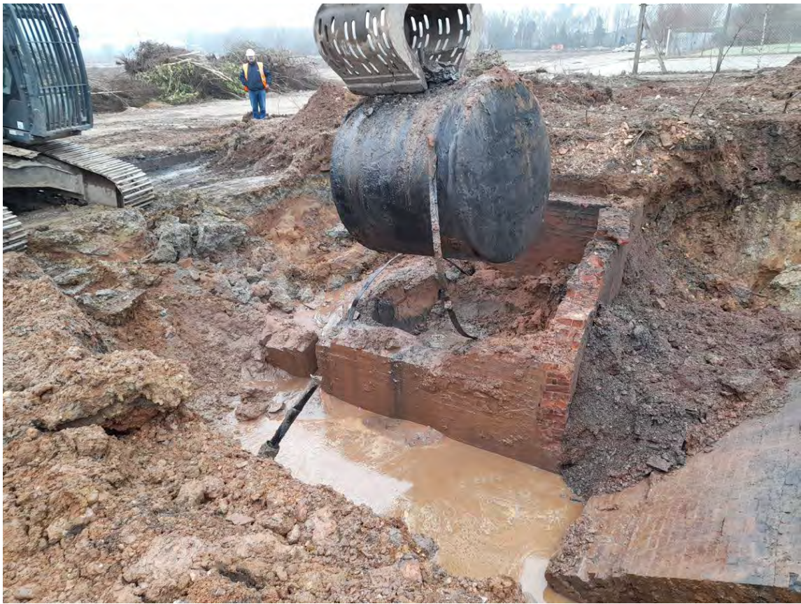
01/03/21 Fuel tank removed from the surrounding brick chamber. The tank was in good condition and showed no signs of leaking
