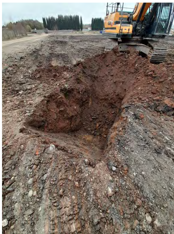
22/03/21 The photo above shows the excavation of validation trial pits around HS2
