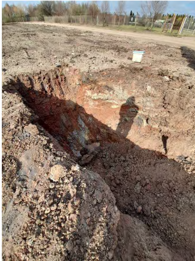
22/03/21 Excavation of validation trial pits around the location of Source 7
