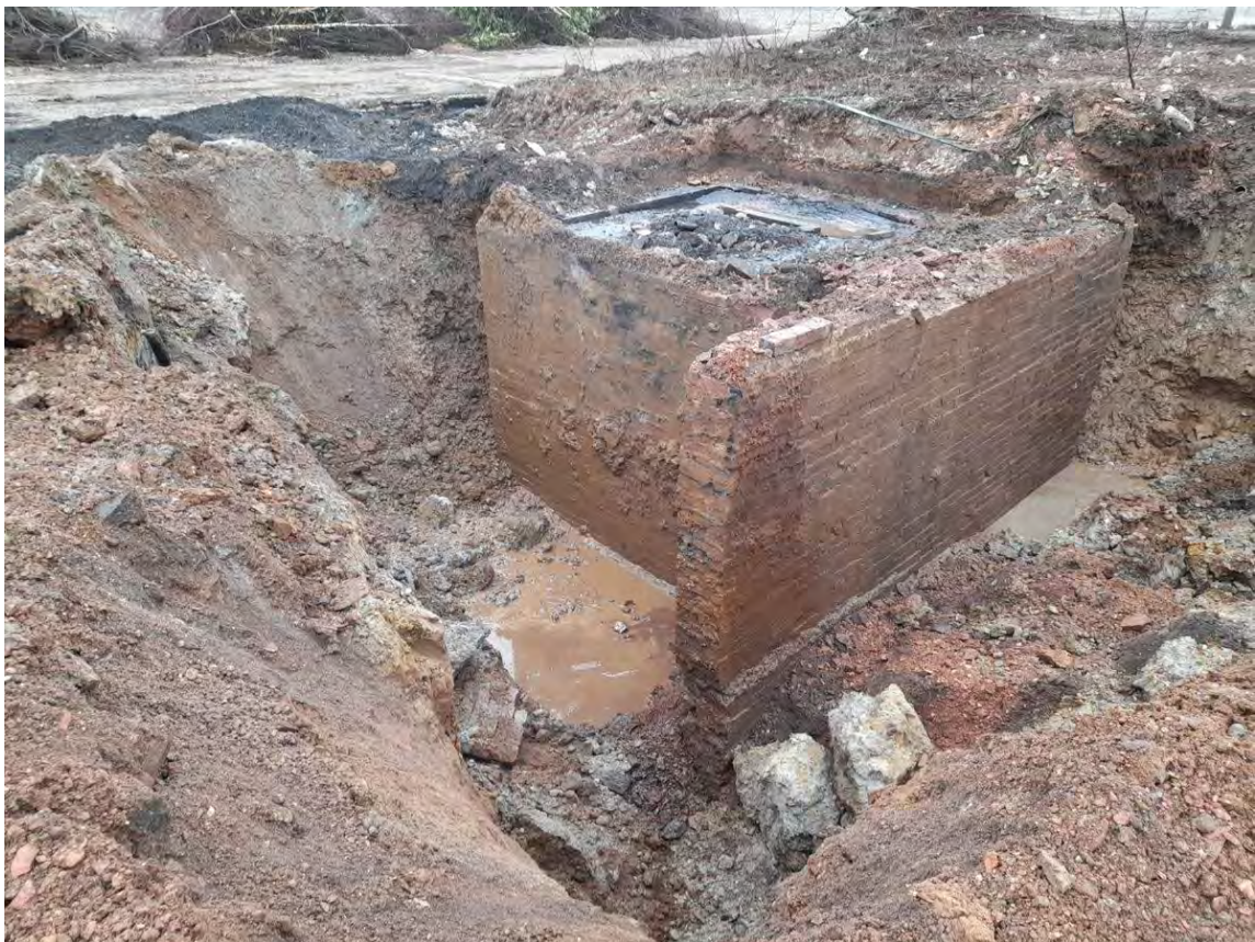
01/03/21 Excavation of fuel tank adjacent to HS1 and validation of the soils surrounding the hotspot
