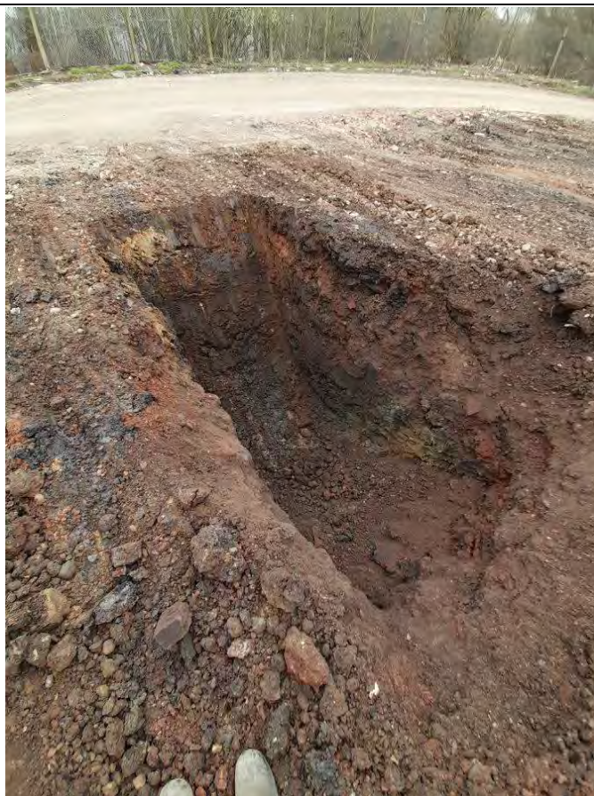
22/03/21 The photo above shows the excavation of validation trial pits adjacent to the retained road infrastructure and HS2
