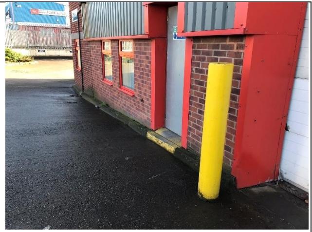
Kerbing installed around building
