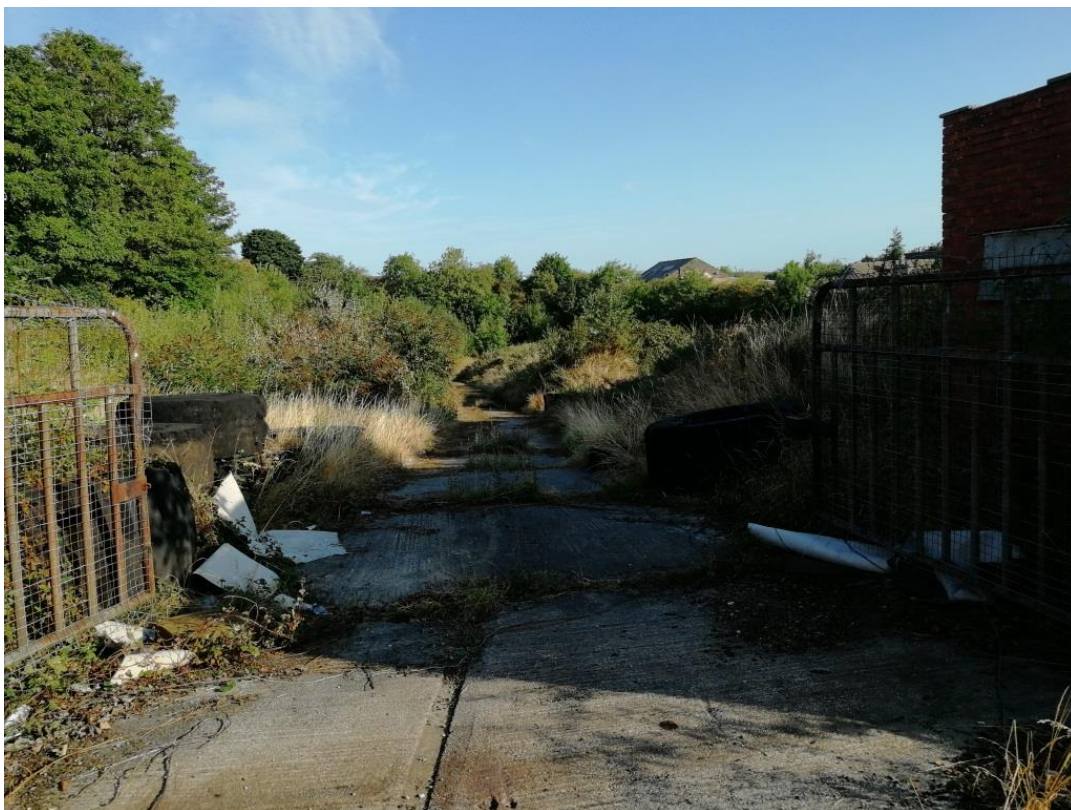
Photograph 4: Ramp sloping north down towards the base of the quarry.
