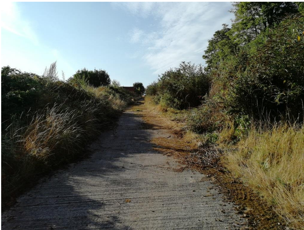
Photograph 6: Half way down the ramp, facing south towards Field Lane.
