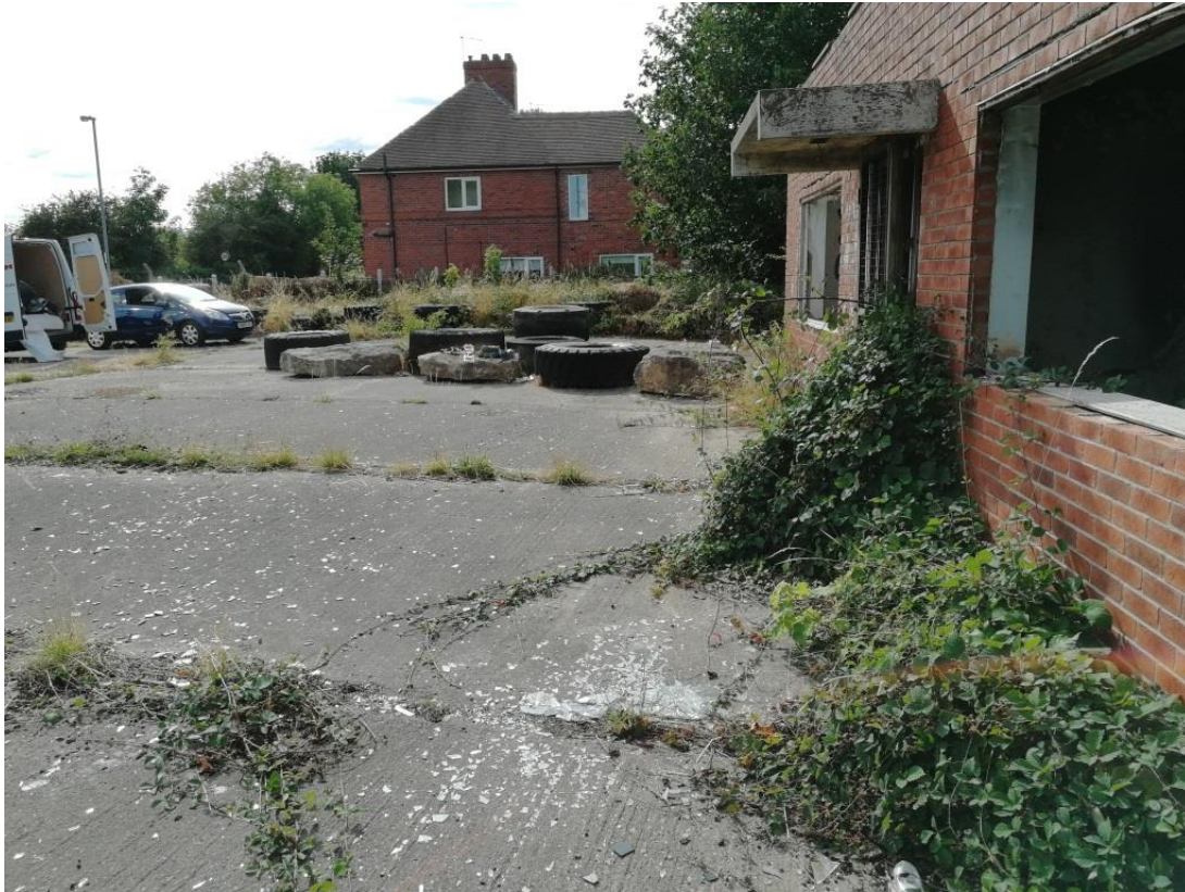
Photograph 3: Dilapidated building in the southwest corner of the site, facing west.
