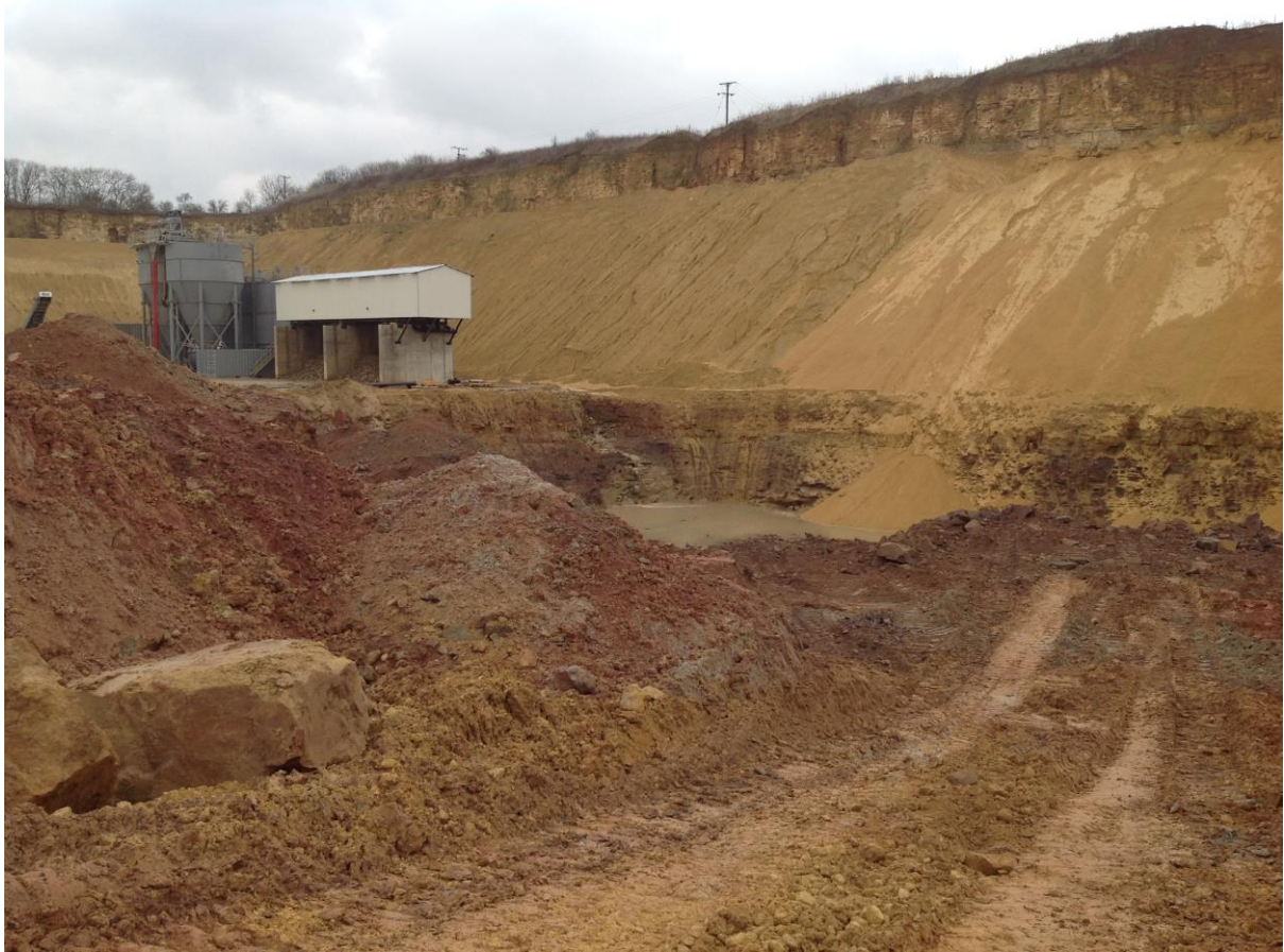
Photograph number 2 showing the temporary quarry sump on the marl excavated in February 2017 near to the wash plant for the quarrying operation to obtain the limestone and use the red marl for the clay lining of the permanent quarry sump.
