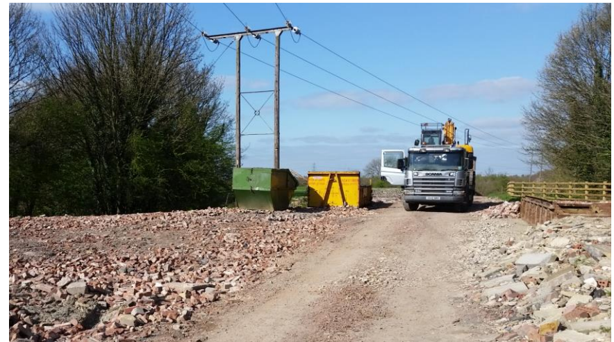
Car park being created and wheel wash installed
