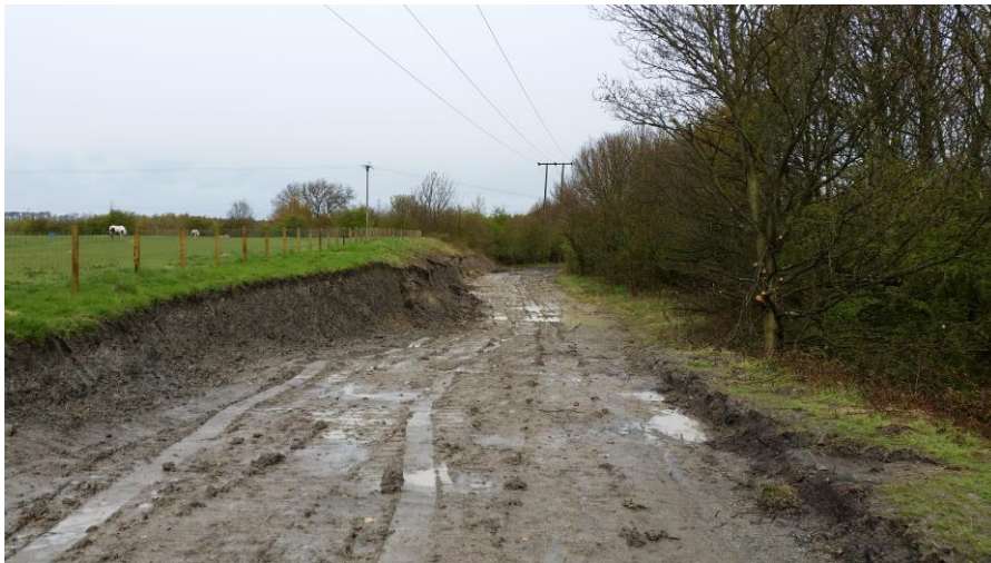
Access Road cut to clear a safe and sight line and pathway under cables
