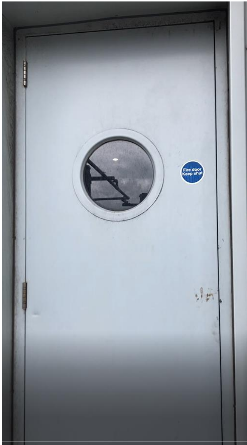
Figure C-2 Containment Testing - Tipping Hall Pedestrian Door
