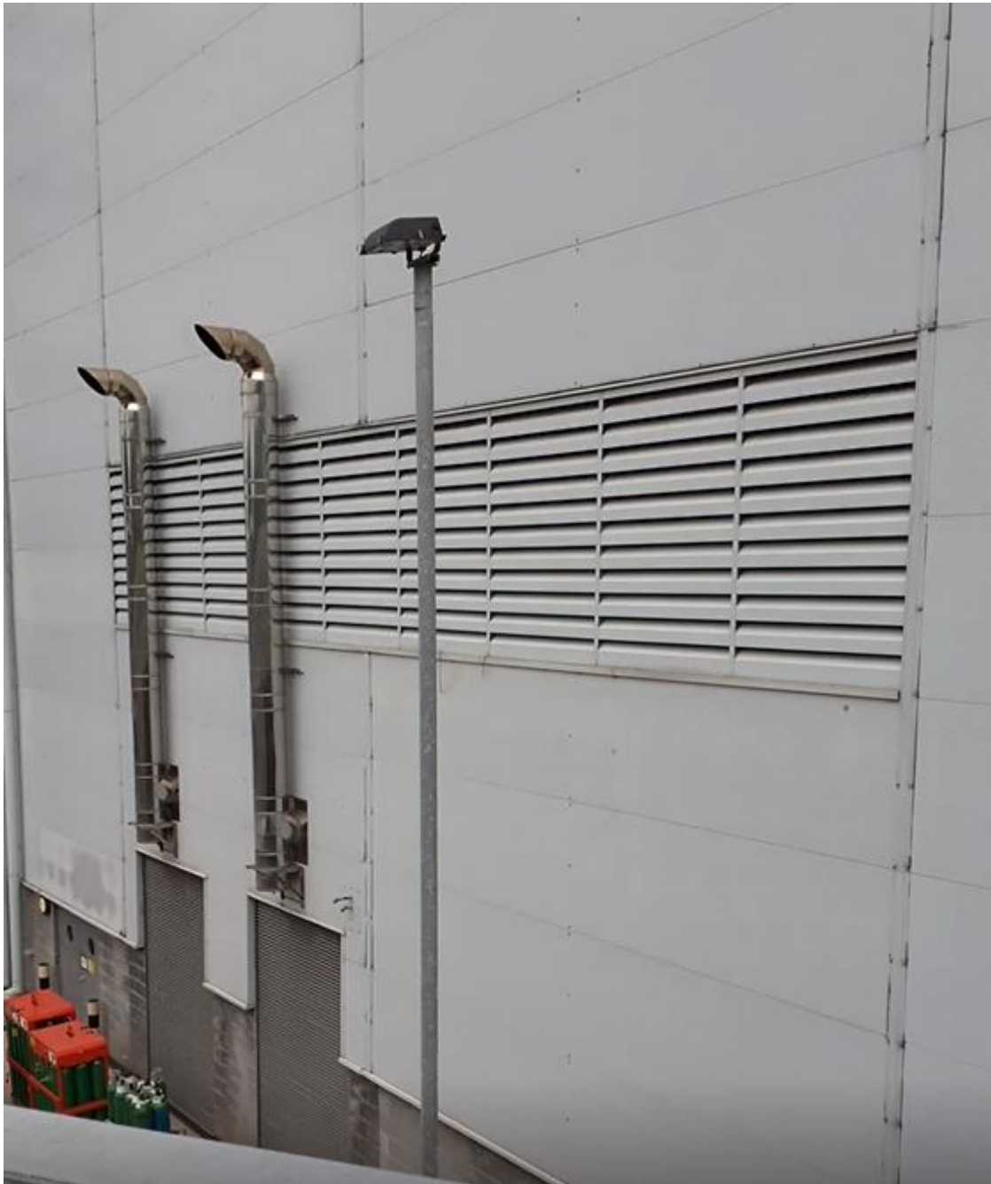
Figure C-1 Containment Testing - Tipping Hall Louvres
