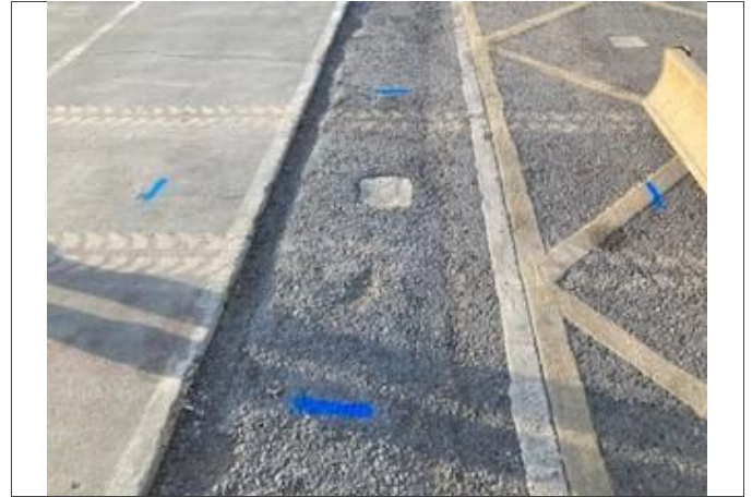
02: 2m box marked for UXO assessment at WS04.
