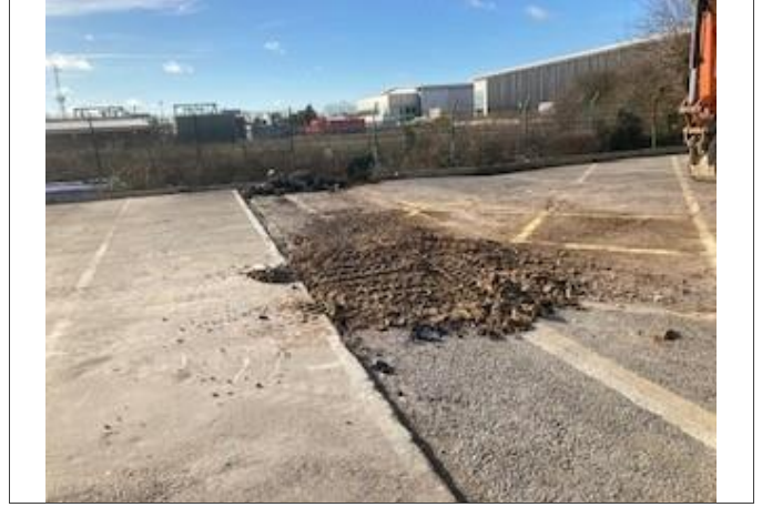
06: Post-con backfilled trial pit.
