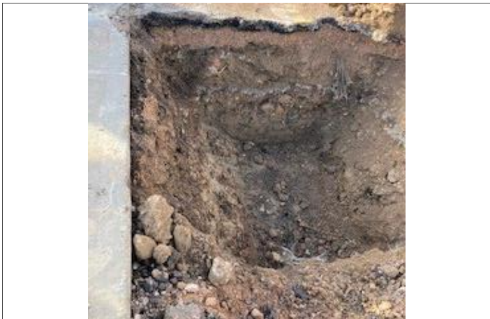
03: The Trial pit exposing granular Made Ground and geotextile membrane.
