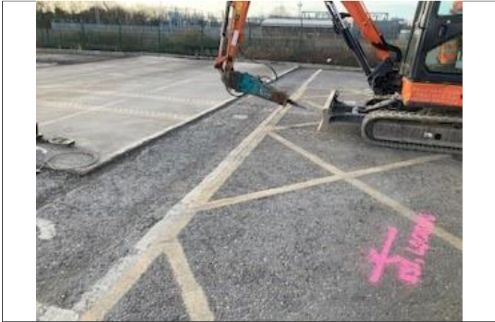
01: Service clearance markings and excavator over WS04.
