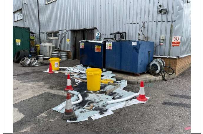
06: ASTs and spill identified at the rear of the building
