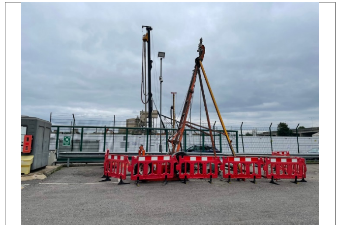
08: Drilling of BH01
