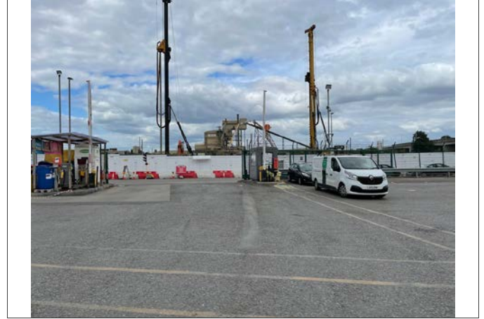
02: Site entrance (north part of the site)
