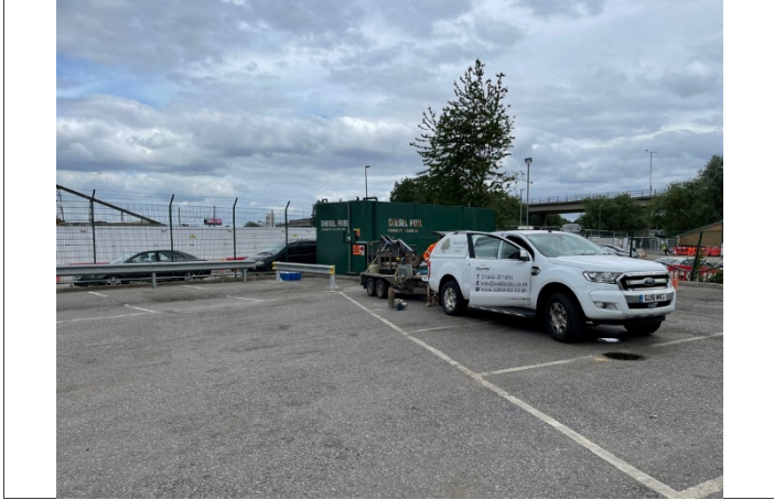
05: Northeast part of the site with associated diesel oil AST in background
