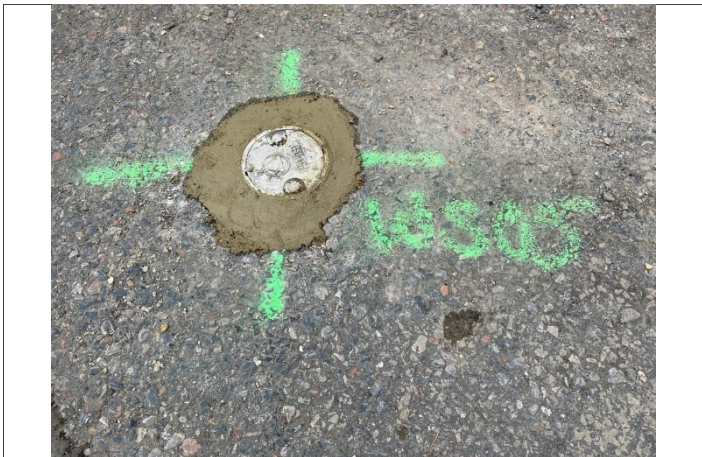
07: Installed monitoring well
