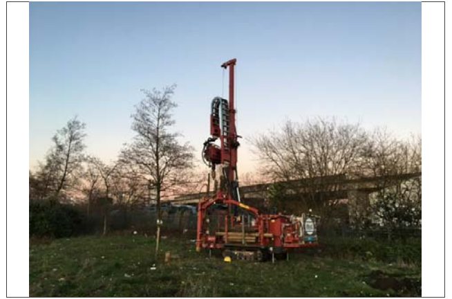
06: Sonic Drilling Rig
