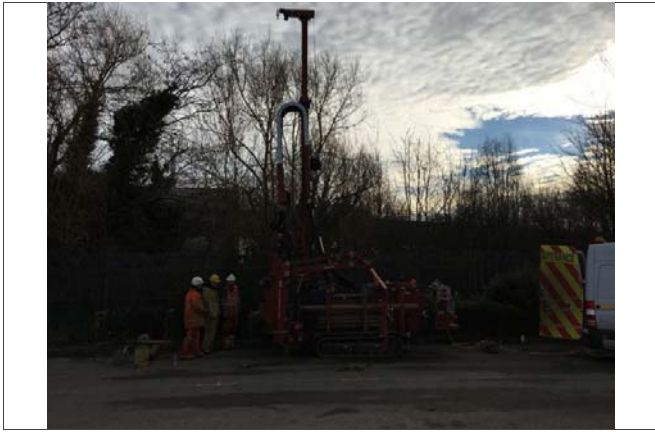
05: Sonic Drilling Rig
