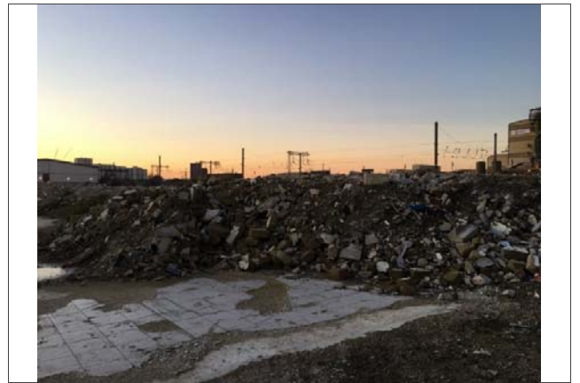
04: Demolition material remaining onsite
