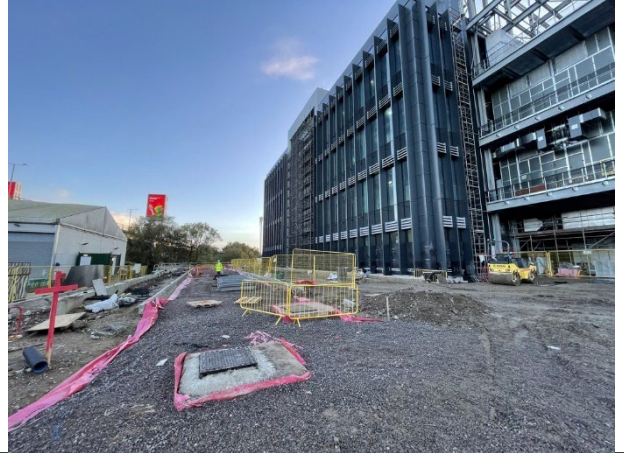
18: Eastern Access Road November 2023
