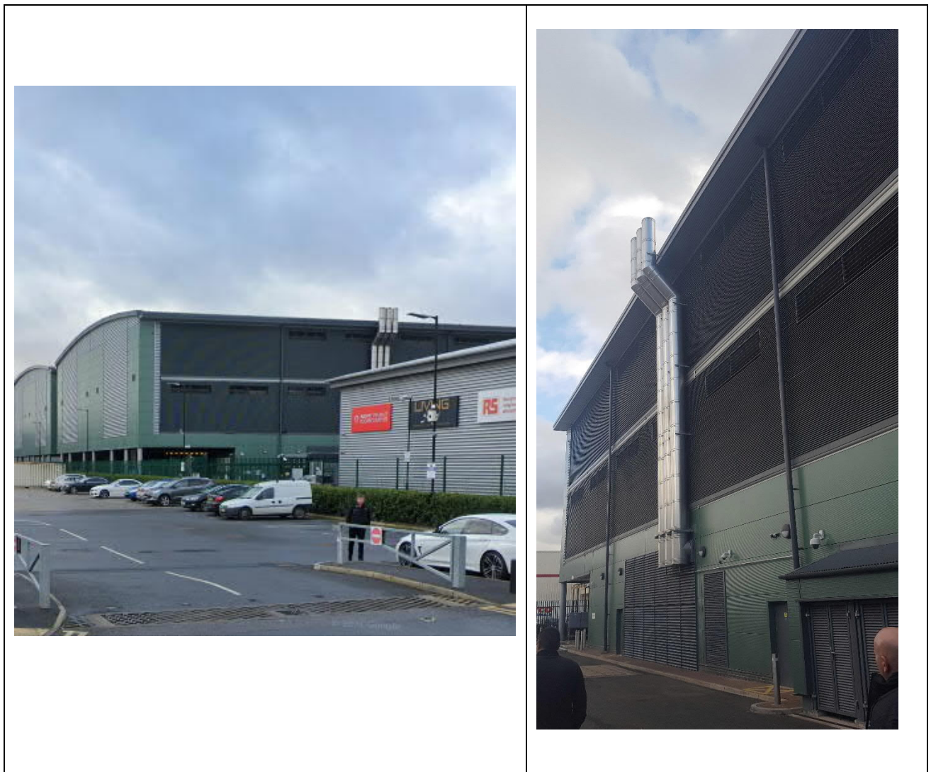
Photograph of existing stack arrangement (3 engine exhausts)
